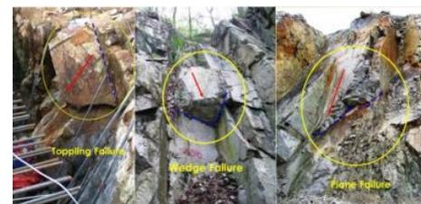
Different Types of Possible Rock Slope Failures
