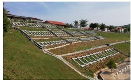
Strengthening of existing slope using soil nails and grid beams
