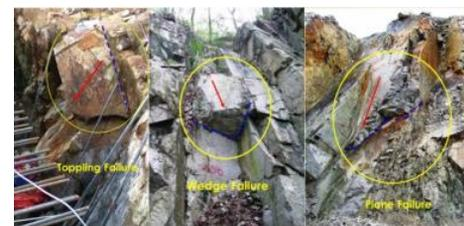
Different Types of Possible Rock Slope Failures
